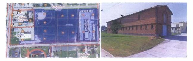
This warehouse building is situated on the southwest panhandle of the parcel. This building has limited electrical service and inadequate lighting. The long narrow lay out and interior columns make use of the space for gross storage less efficient that other arrangements might provide.
